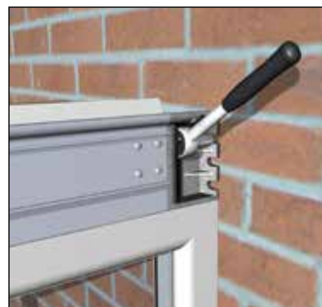
Where the eaves beam sits against the host masonry wall, it has a structural moulding attached to the eaves beam. This has three fixing positions cast into it to allow attachment into masonry – choose the hole that directly lines up with solid masonry and attach using one resin anchor suitable for substrate / loads (not supplied, see p21 Appendix 1).
