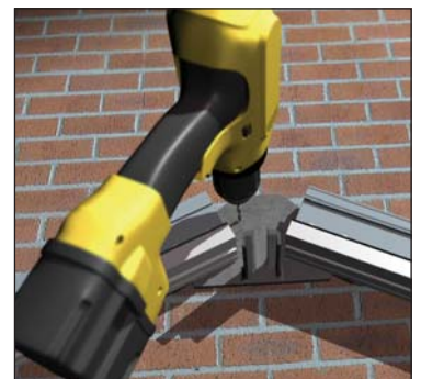
The ridge hanger/compression plate is attached to the host wall using two anchor bolts (supplied).
