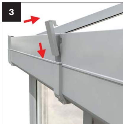
Slide the bracket into place ensuring bracket cleats slot into the top Cornice section.
