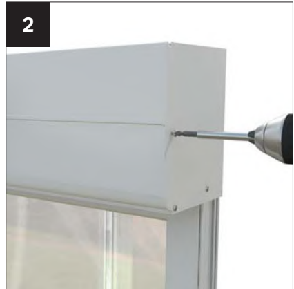
2 GUTTER STOP END DETAIL - Used with lean-to roofs, gable roofs or when then gutter returns along the host wall. Secure the end plate into position using the fixings provided (CRN008).
