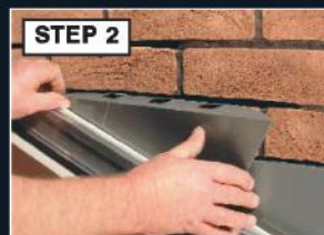
Start installing Conservaflash™ from gutter end towards the ridge
