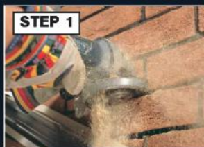
Chase out with grinding wheel
