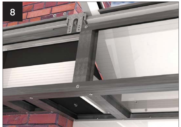
8 Fix the vertical frames in place using CHA006 (bag of 25) as per standard installation.
