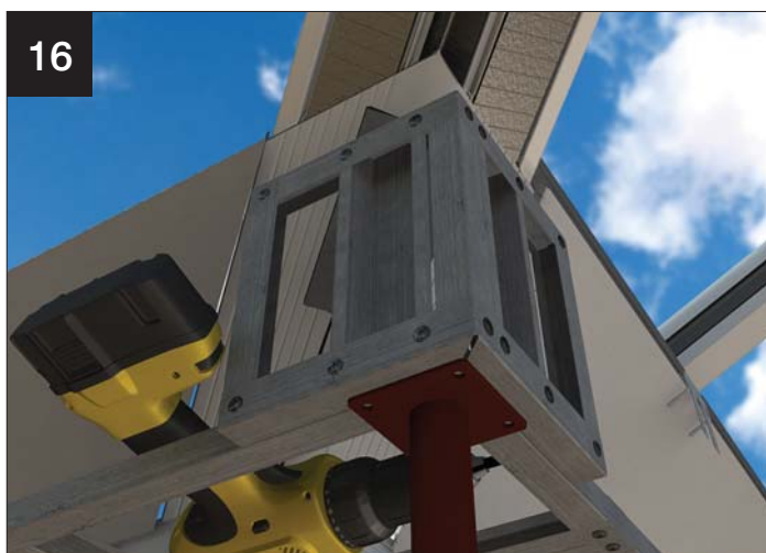
Valley infill panel fitted to horizontal frame, as image 10
