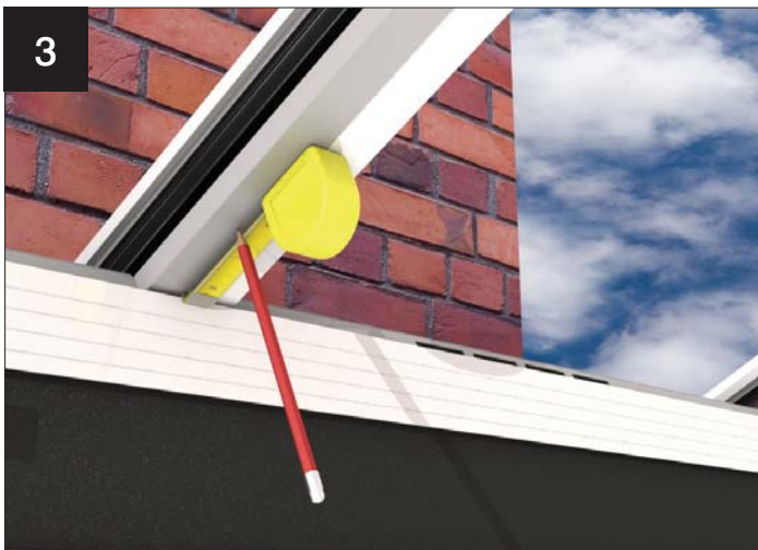
3 Using LHE---/2 as a datum, measure and mark the positions of the brackets in line with the dimensions given in the provided paperwork.
