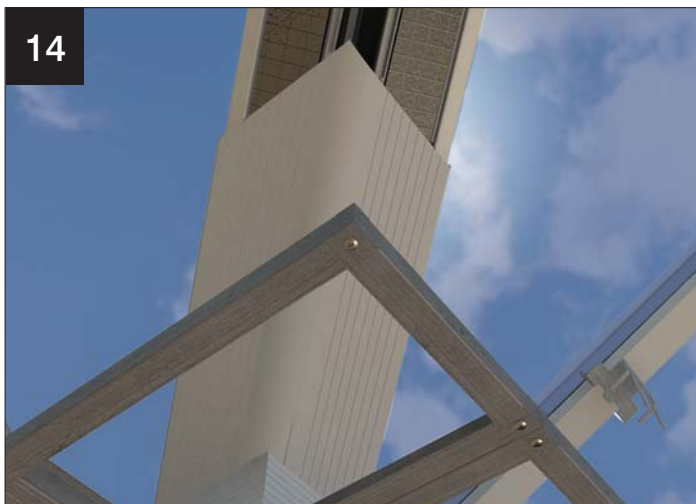
Measure and fit the standard valley undercladding NVU-V between the eaves and mark 'C'. Scribe to suit.
